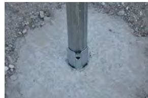
Flexible/Bending Sign Support
