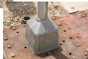
Cast Aluminum Luminaire Support
