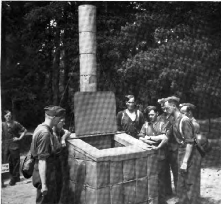
PLATE VI: Army School of Hygiene. A Bailleul Incinerator built of Earth-filled Petrol Tins
