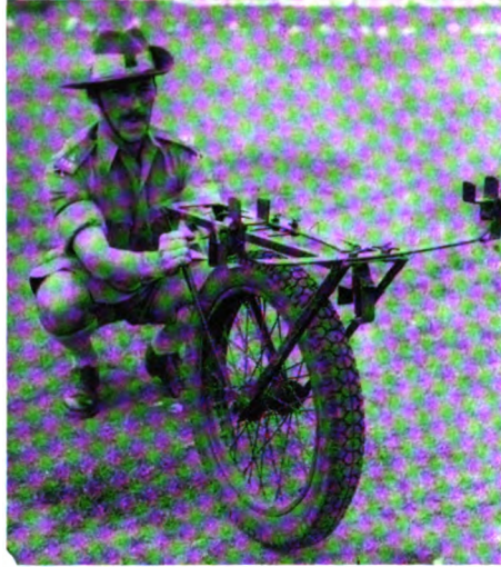
PLATE XVIII. 2nd Division. One wheeled folding stretcher-carrier.
