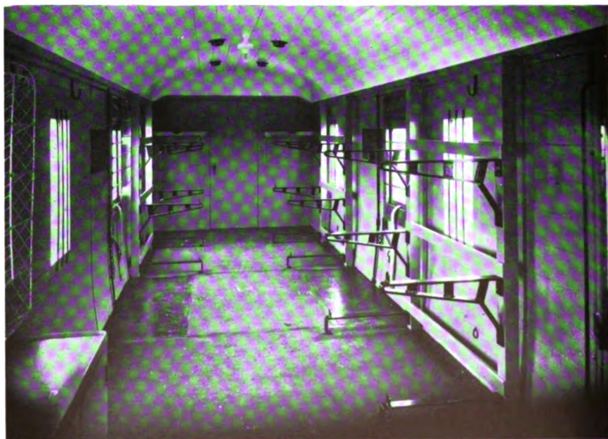
PLATE XXIX. L.M.S. brake van fitted for stretcher cases
