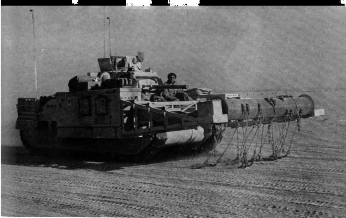
4. A Scorpion; Matilda tank with flails to destroy mines.
