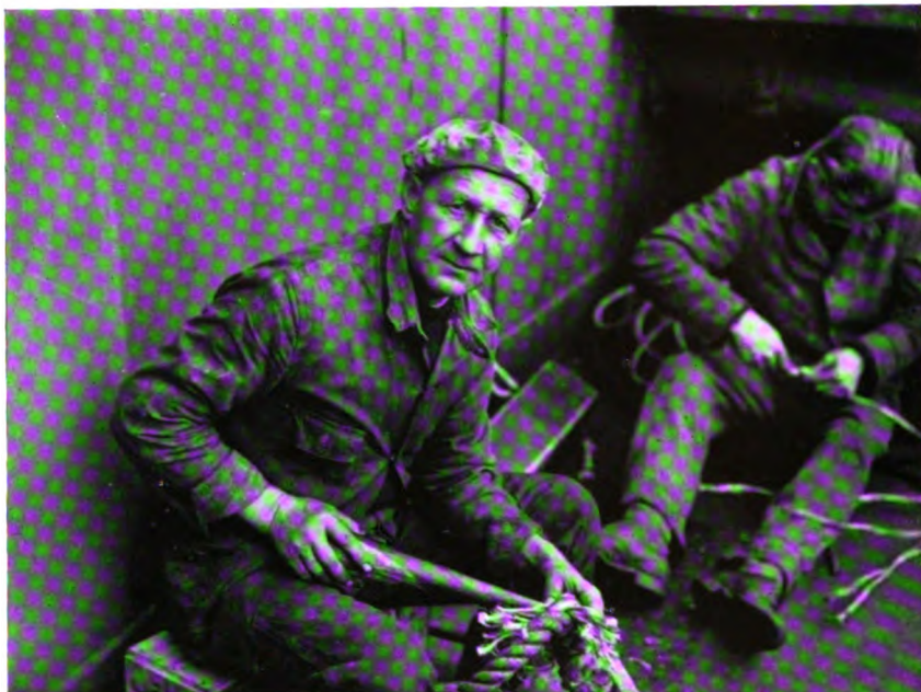
Splicing a rope
