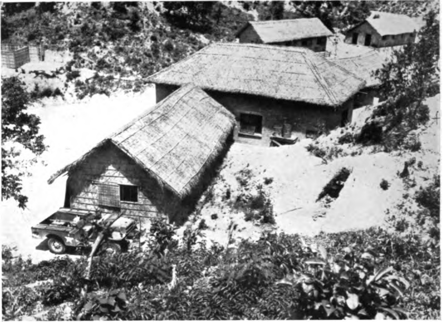
PLATE XXXV. No. 63 M.F.H., general view of 'Basha' type wards.
