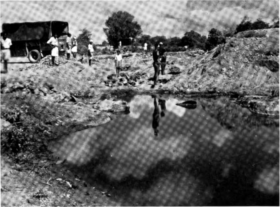
PLATE XLIII. Man-made malarial hazard. Water collecting in a borrow pit.
