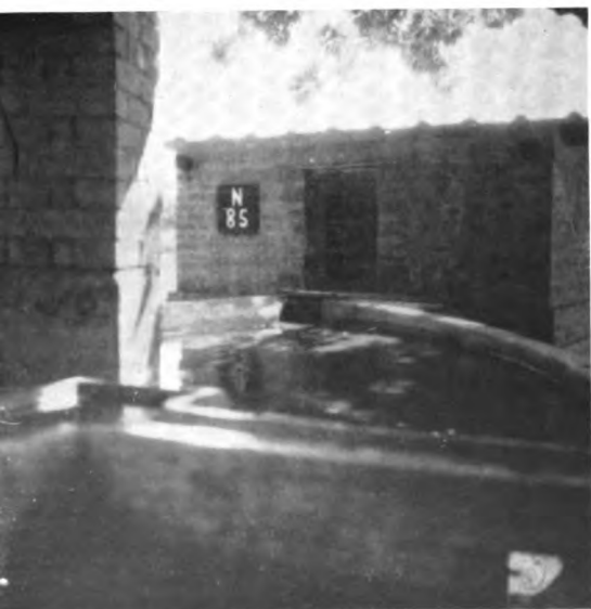
PLATE LXII: (3) Open storage tank
