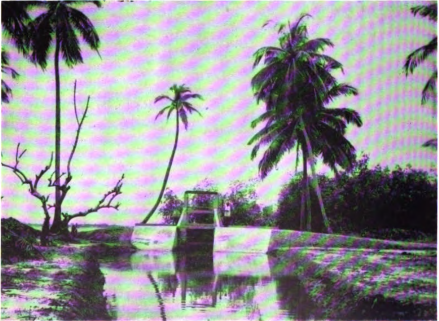
PLATE XXXV: Anti-malaria measures. Tidal gate in bund controlling the system
