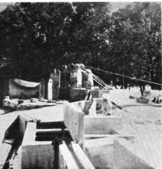
PLATE LX: Water supply at Phaphamau. (1) Dhobi ghat
