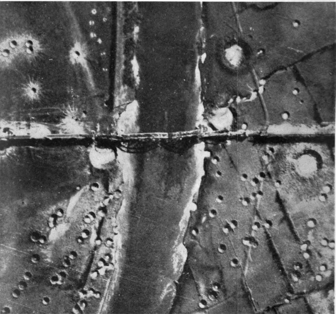
24. Nienburg Bridge after the attack on 22nd March 1945, showing Grand Slam craters.
