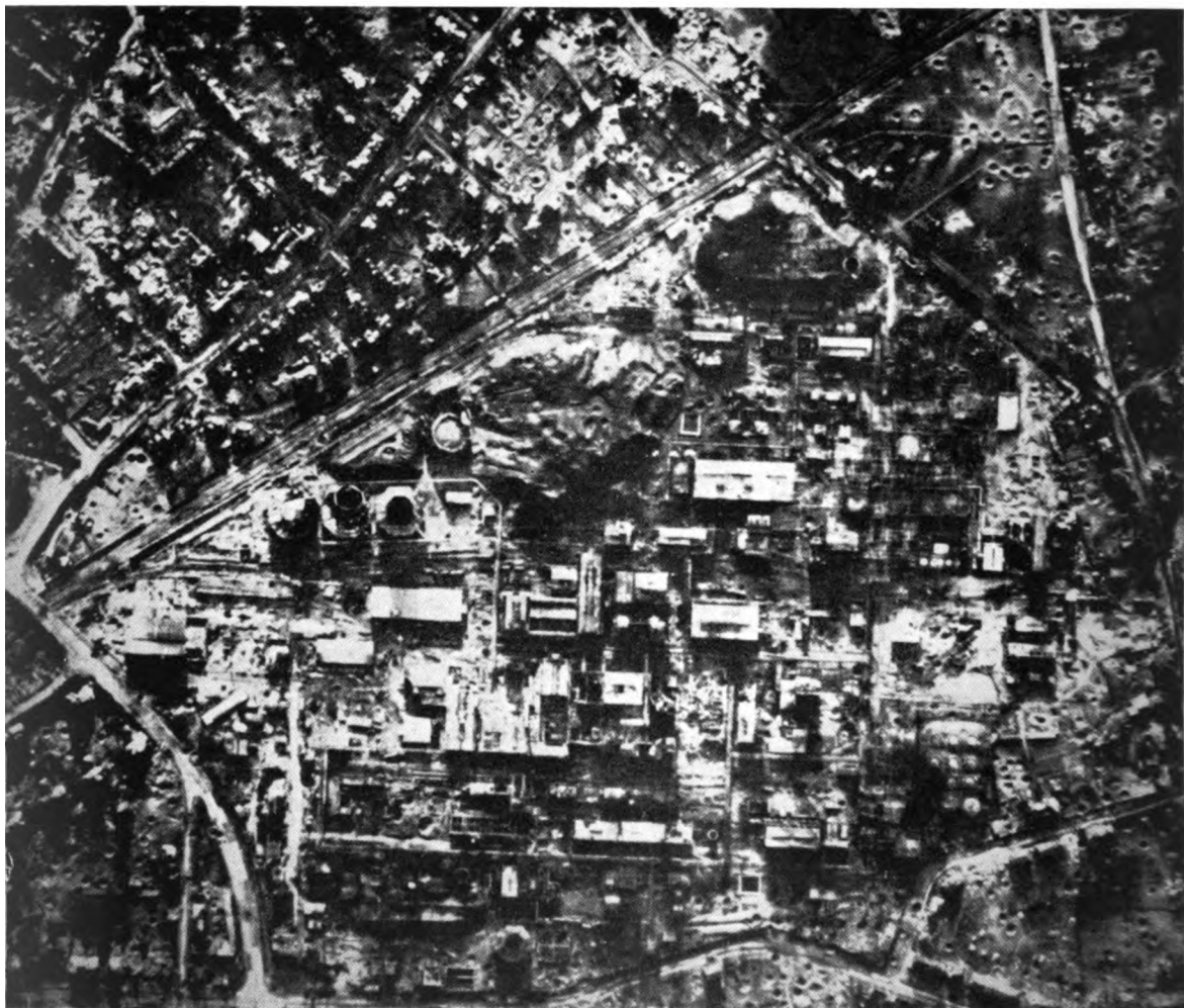
12. The oil plant at Bottrop/Welheim on 18th November 1944 after attacks by Bomber Command and the United States 8th Air Force.
