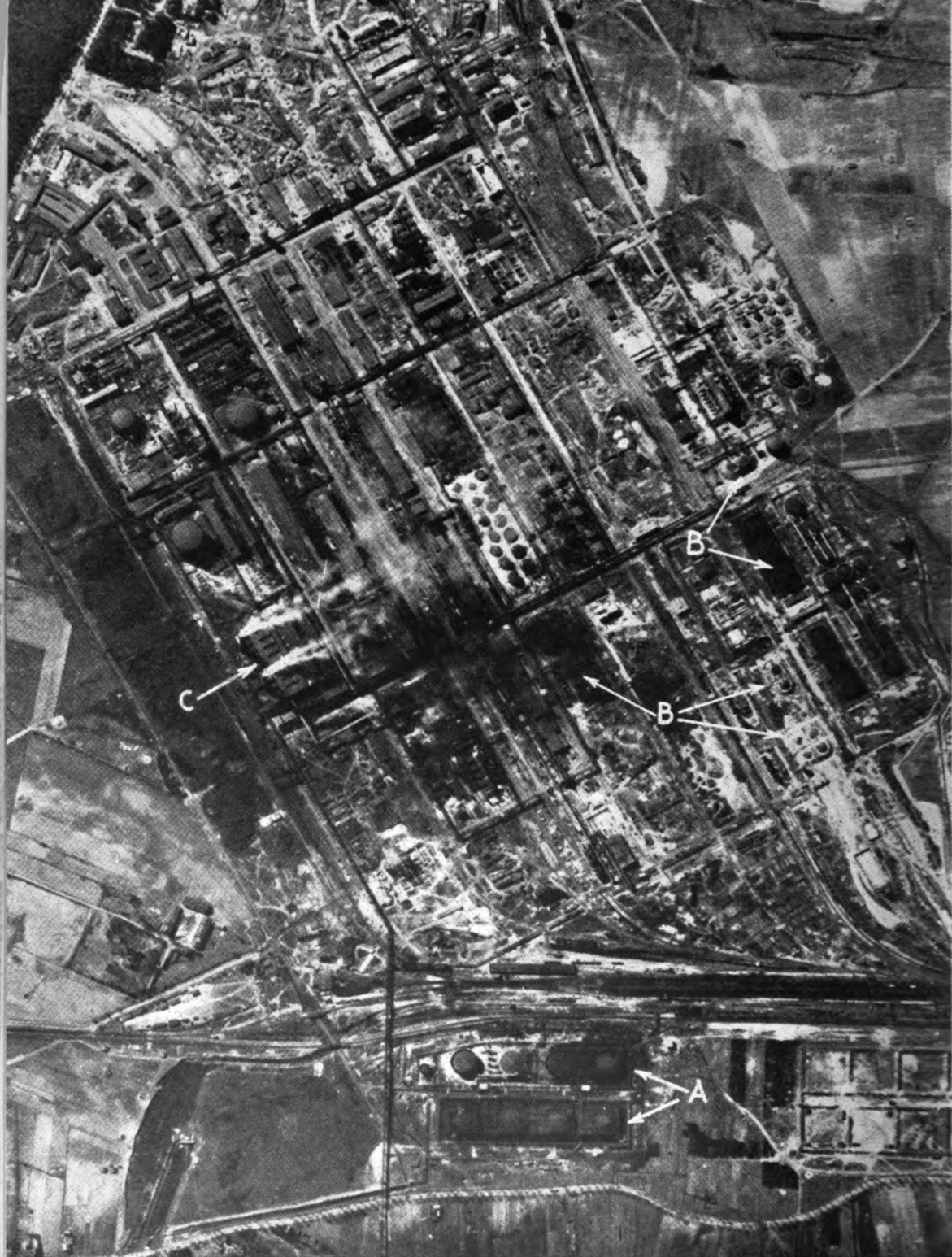
20. The oil plant at Pölitz before attack.
