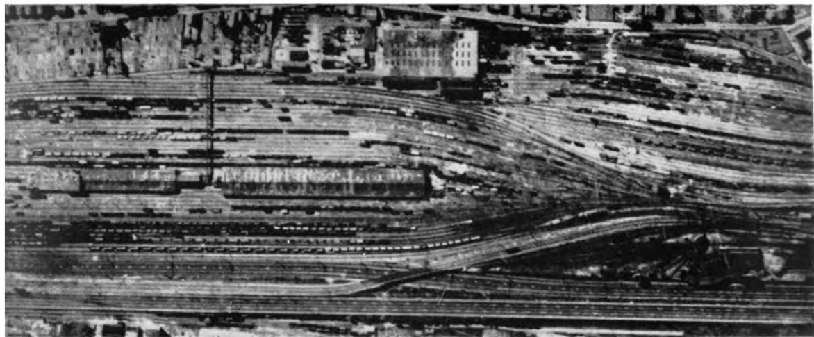
2. The marshalling yards at Juvisy before attack.
