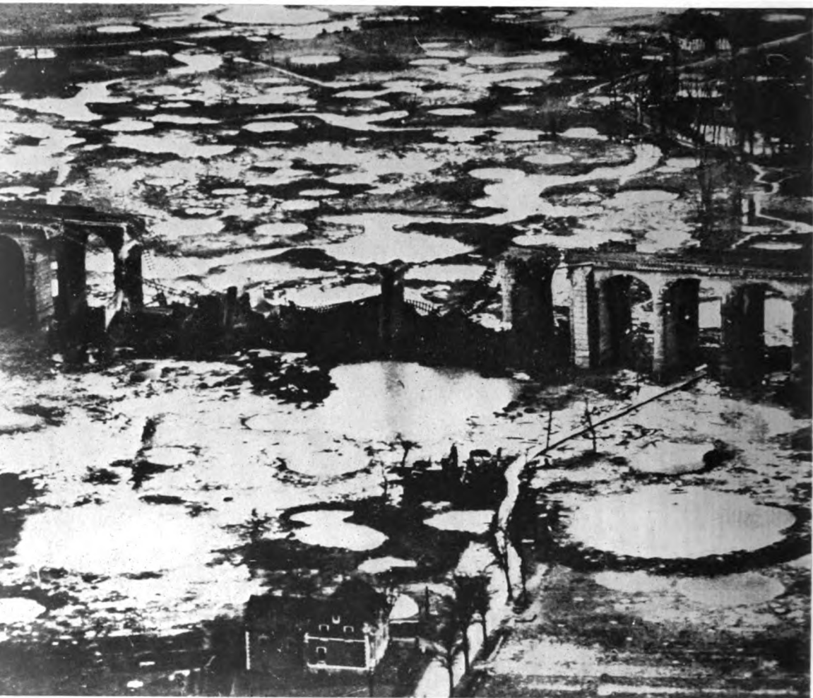
22. The Bielefeld Viaduct on 17th March 1945.
