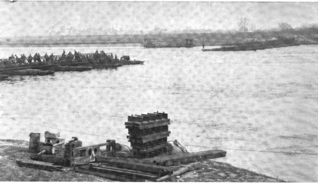
47. Bridge over the Rhine being built
