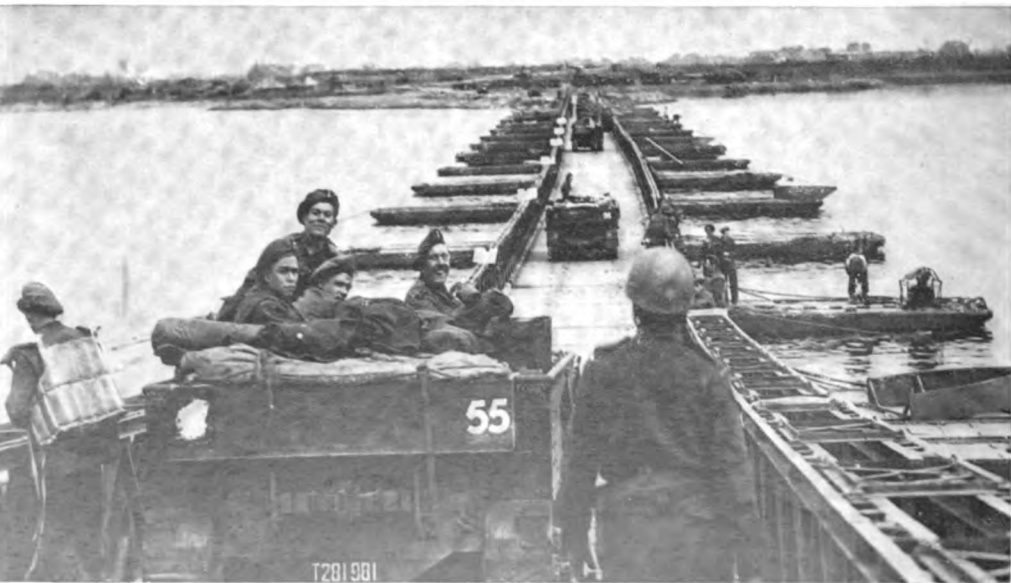
48. Completed bridge in use
