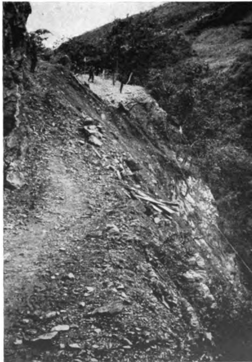
39. The Tiddim road blocked by a landslide probably caused by bombing.
