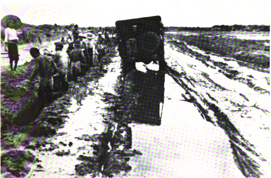
3. Trying to clear floods at Pegu airfield, May 1945.
