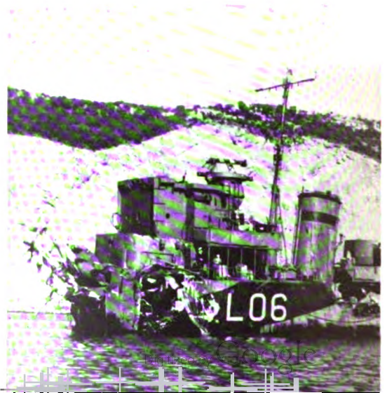
The Hunt-class destroyer Avon Vale , showing damage caused by air torpedo off Bougie, 29th January 1943.
