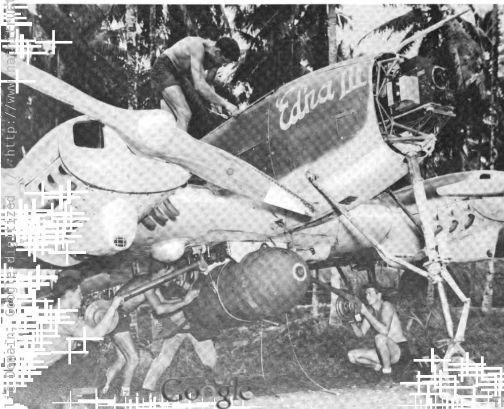
A TDR-1 is prepared for an attack somewhere in the Pacific. Note the television camera in the nose.
