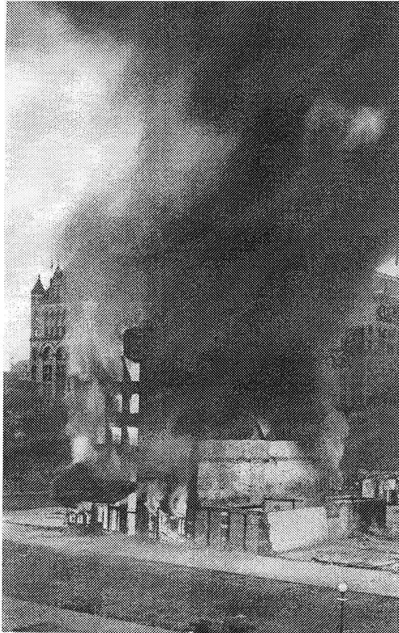
Fig. 4. Burning test buildings near the corner of 10th and B Streets, NW, in Washington 10 to 20 minutes after ignition on Sunday morning, June 17, 1928. These burning buildings are on the present day site of the Justice Department Building. The Old Post Office building is in the background. (Used with permission of NFPA.)
