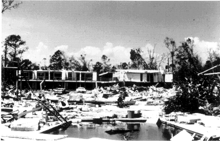
Fig. 3. Damage to buildings due to hurricane winds (Hurricane Camille, August 17, 1969).
