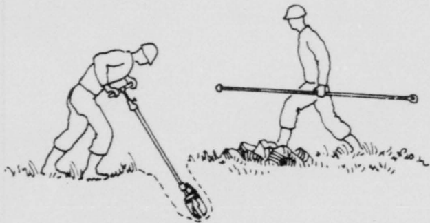
TEAM ONE: 120 Minutes—Dig anchor holes and install anchor rods and anchor plates for Anchor Bridles I and II (see page 35).
