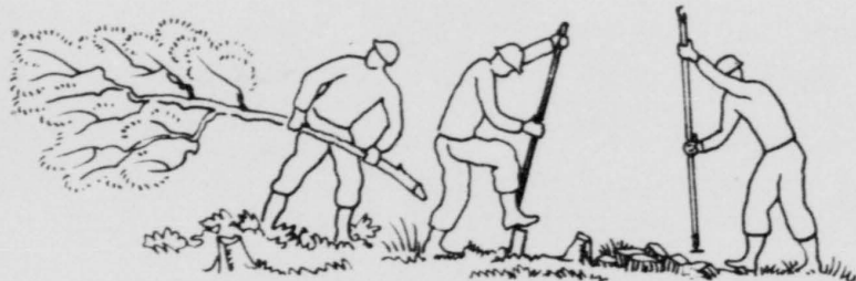
TEAM ONE: 60 Minutes — Fill up and tamp remaining holes, clear ground, prepare camouflage, etc.
