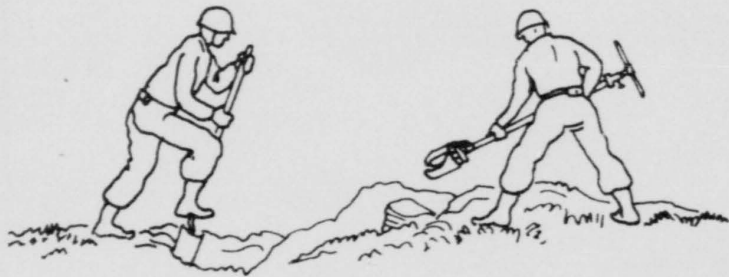
TEAM ONE: 150 Minutes — Dig holes and install anchor rods and anchor plates for Masts I and II (see page 35).
