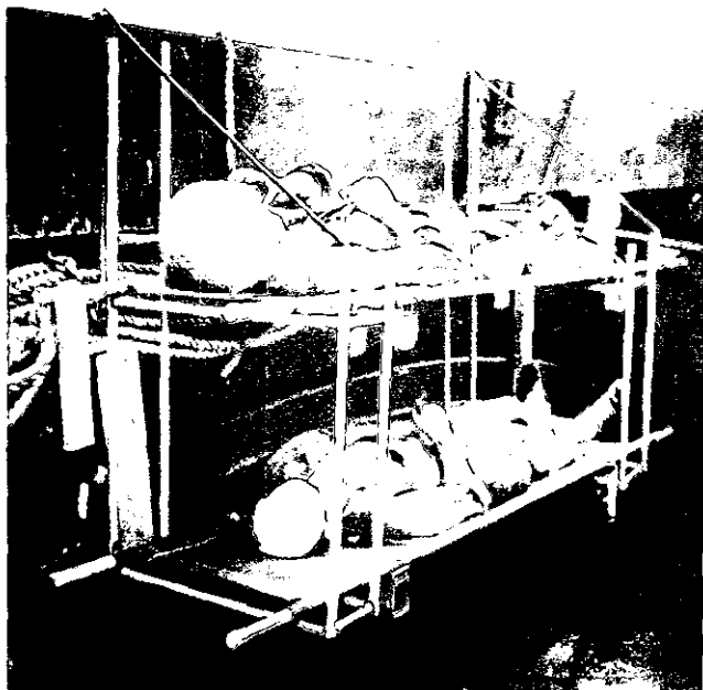
Figure 214. Improvised litter racks on small landing craft (Australian maneuvers).
