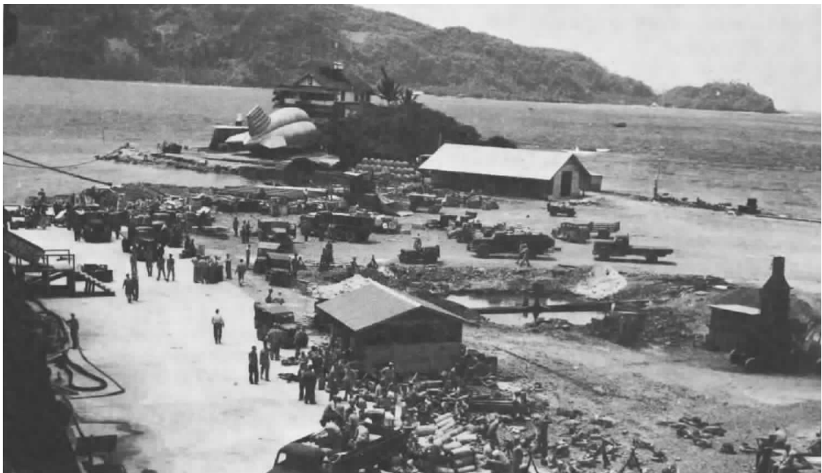
Barrage balloon in background ready in case of air attack on unloading area. (USMC Photo 51110)
